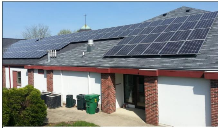
Solar panels on Englewood Christian Church, an evangelical Christian church on the eastside of Indianapolis. Photo provided by Creation Cares Partners
